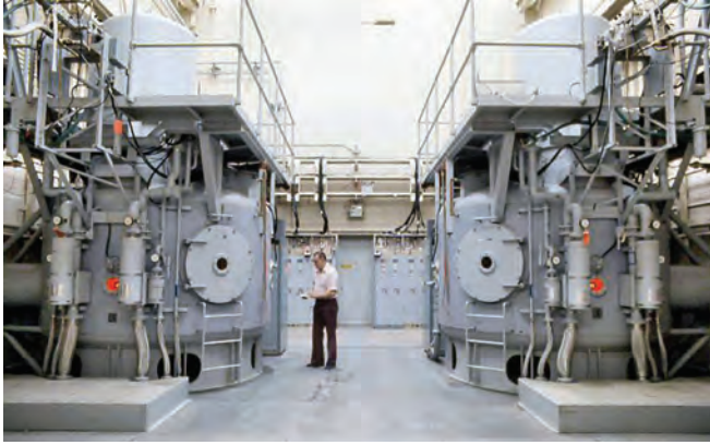
Historic photo showing the Klystron tanks. This photo is taken from the opposite end of the room to the previous one. Provided by Clint Esciklsen
